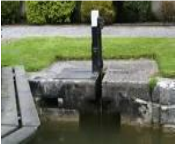
1. Ratchet Mechanism for a Ground Paddle
